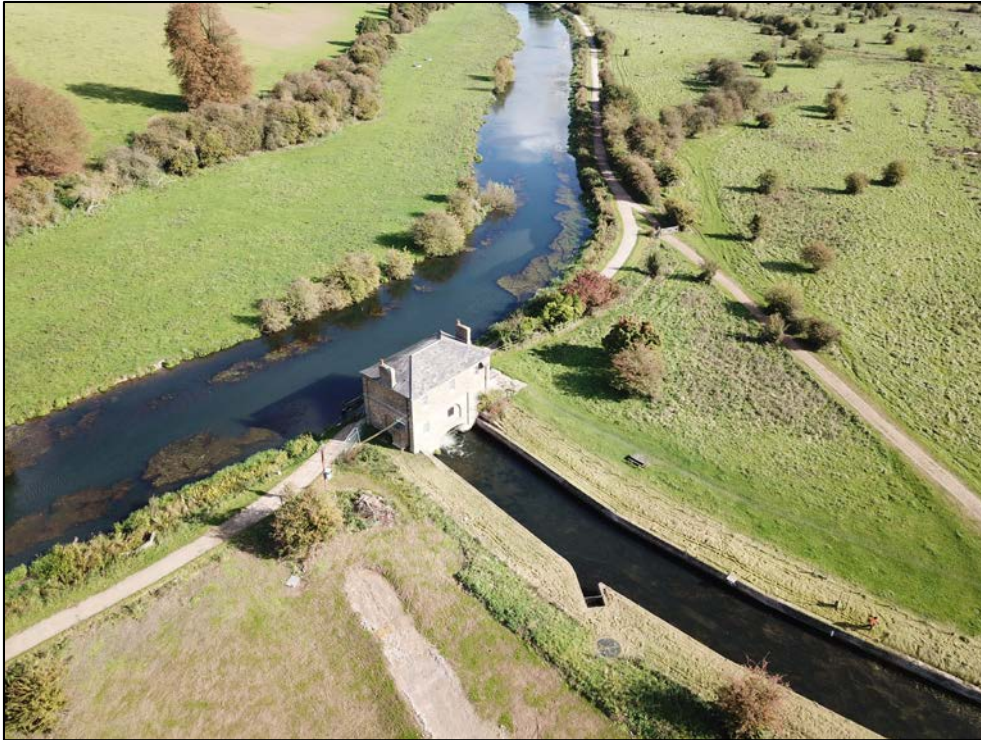
Figure 1. The Drone image illustrating New River and Gauge house that built.
