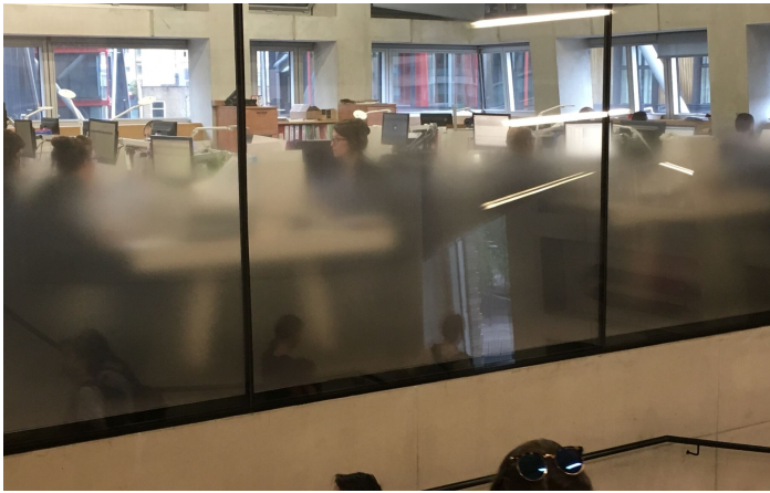
Fig. 10. Public view of offices from the Switch House staircase.
