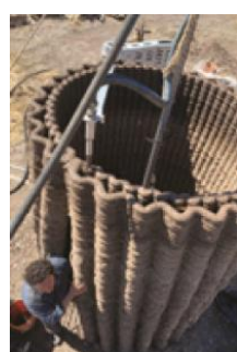
Figure 6-7-8. On-site 3D printing of Tecla[12] photo credit: WASP, Casa Covida[11], photo credit: Emergent Objects and Tova[13], photo credit: Gregori Civeru.
