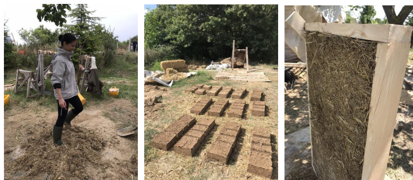
Figure 1-2-3. Traditional earthen building methods such as cob and adobe are labour intensive and slow.
