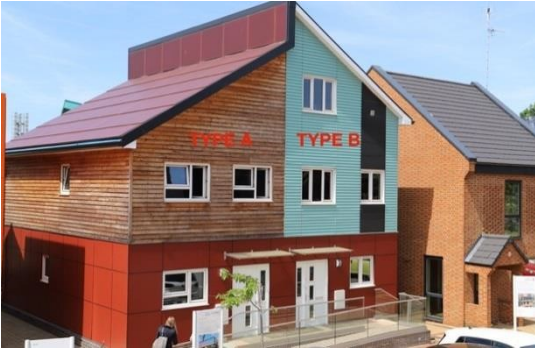
Fig. 1. The case study building.
